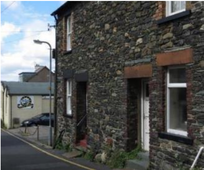
North east side of Standish Street. The red lintels are Penrith sandstone.
