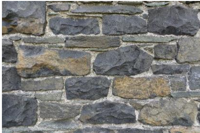
The darker blocks in this wall are Castlehead dolerite that have slightly irregular surfaces in contrast to the lighter coloured blocks with flatter faces of material from the Borrowdale Volcanic Group.
