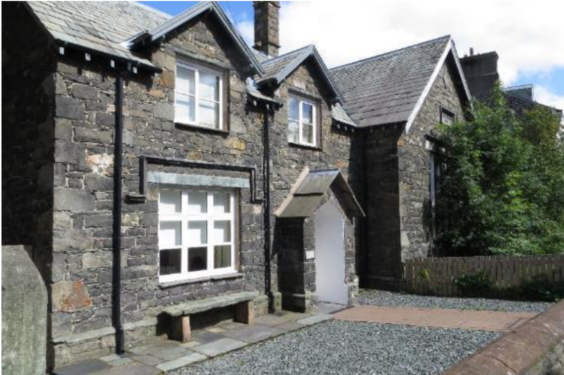
Most of the blocks used to build Vergers Cottage on St John's Street are Castlehead dolerite.
