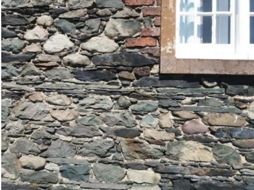
Gathered stone in the front wall of St Herbert's Centre, High Hill
